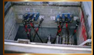
Manufactured to ANSI/IEEE Standard 386 Vault Installation using 6 Point Stacked Style Junction Bars
